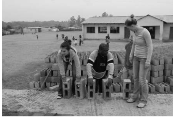
Moving Bricks Closer to the Foundations
